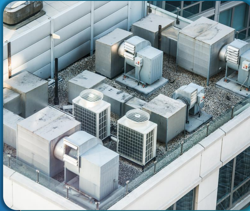
Commercial Combustion Water/Space/Heating/ Cooking/Others
