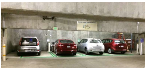
Figure 3: Getty Center parking structure, Level 2 EVSE
