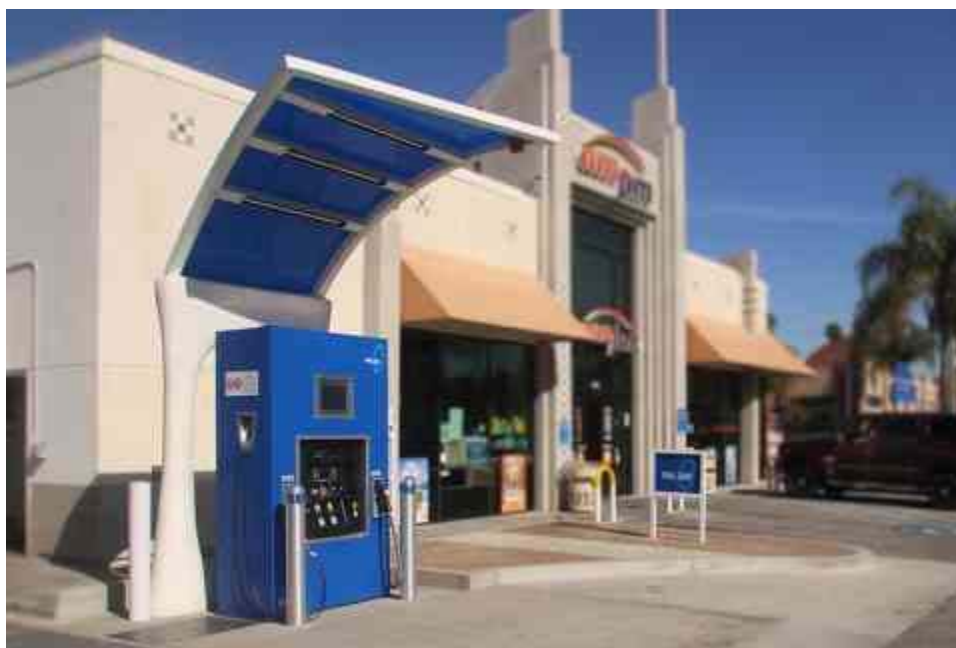
Figure 25: FirstElement Retail Hydrogen Station Co-located at ARCO Gas Station in Long Beach
