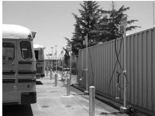
Figure 1: Time-Fill Posts Allows Beaumont USD to Fill 8 Buses Overnight
