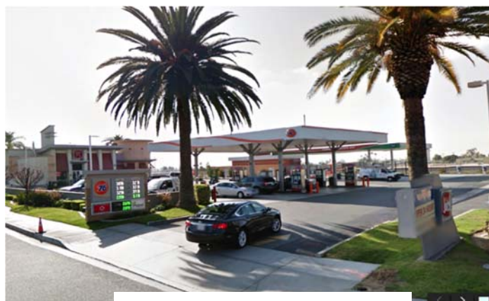
Figure 19: Ontario CNG Station
