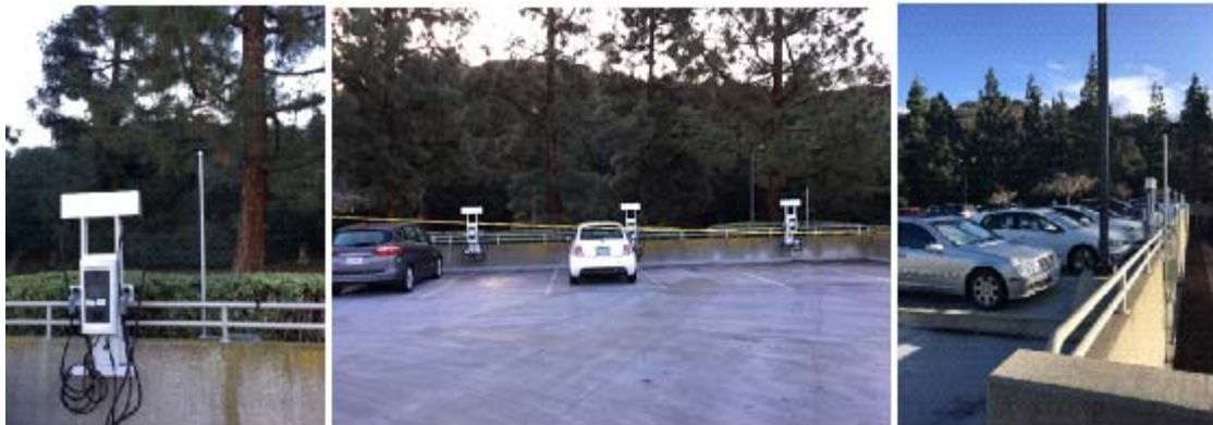
Figure 32: Installations in Progress
