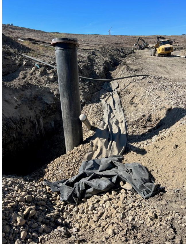
Figure 5 - Leachate Seep Remediation – north edge of reaction area.
